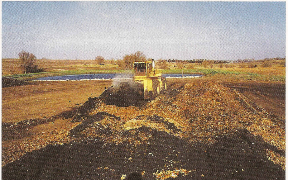
Biosolids come in from the treatment plant everyday, and are mixed with grass, leaves and woodchips.
